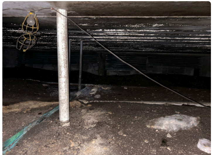
Condensation in crawlspace
