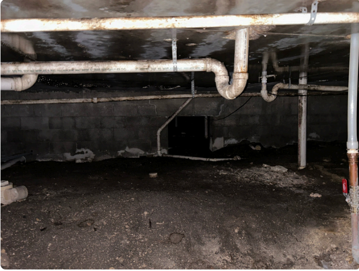
Condensation in crawlspace
